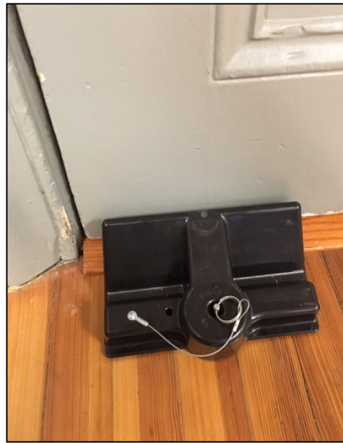
4. Door is now secured.
